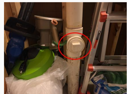
Inside the basement closet
