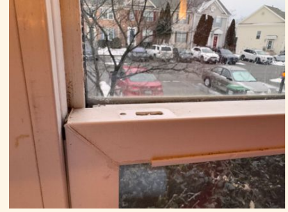
Broken tilt latch
