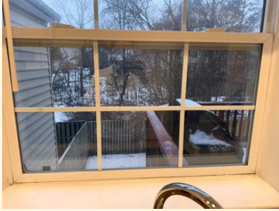
Kitchen window sealed shut with caulking
