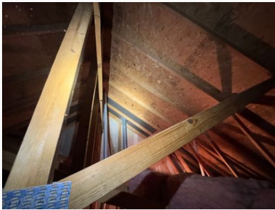
Pictures of roof structure
