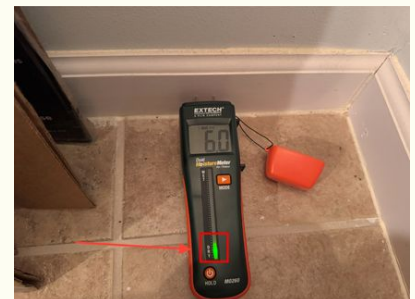
Dry at the time of the inspection
